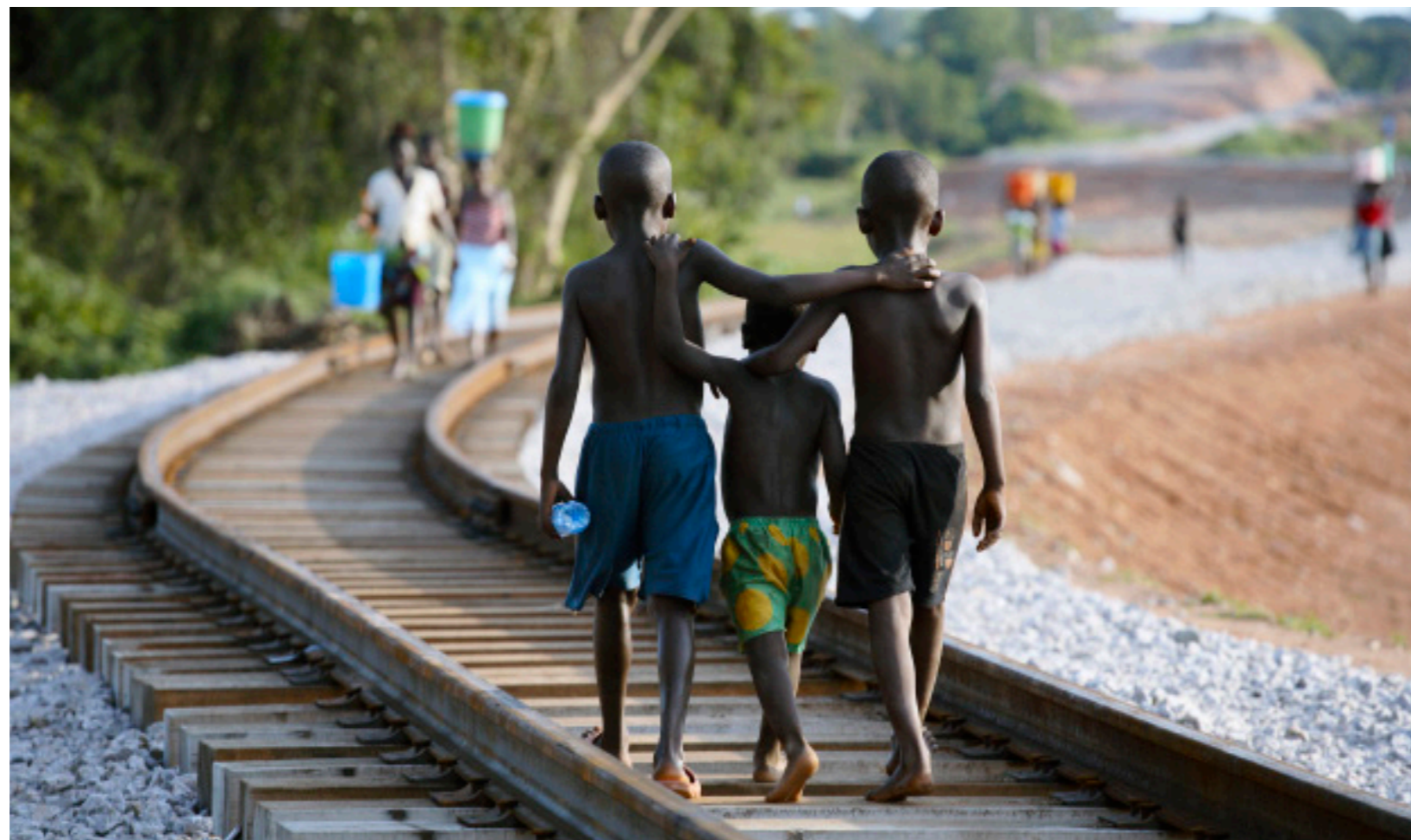
Above Boys walk on newly-laid railway tracks in Dondo, Angola. The country has used profits from the oil boom to rebuild its infrastructure
